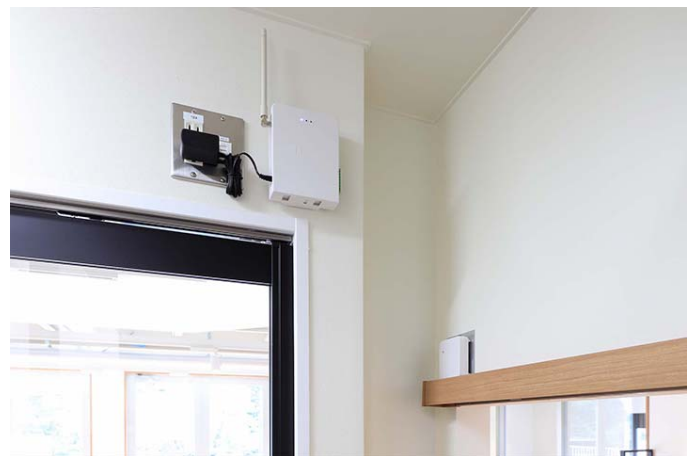
In-kitchen relay unit (left) and a temperature/humidity sensor (right).
