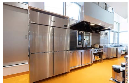
All kitchen equipment, including refrigerators and combi ovens, are Fujimak products.
